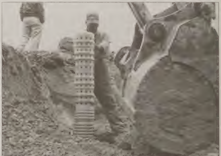
Grade Stabilization using a Hickenbottom device
